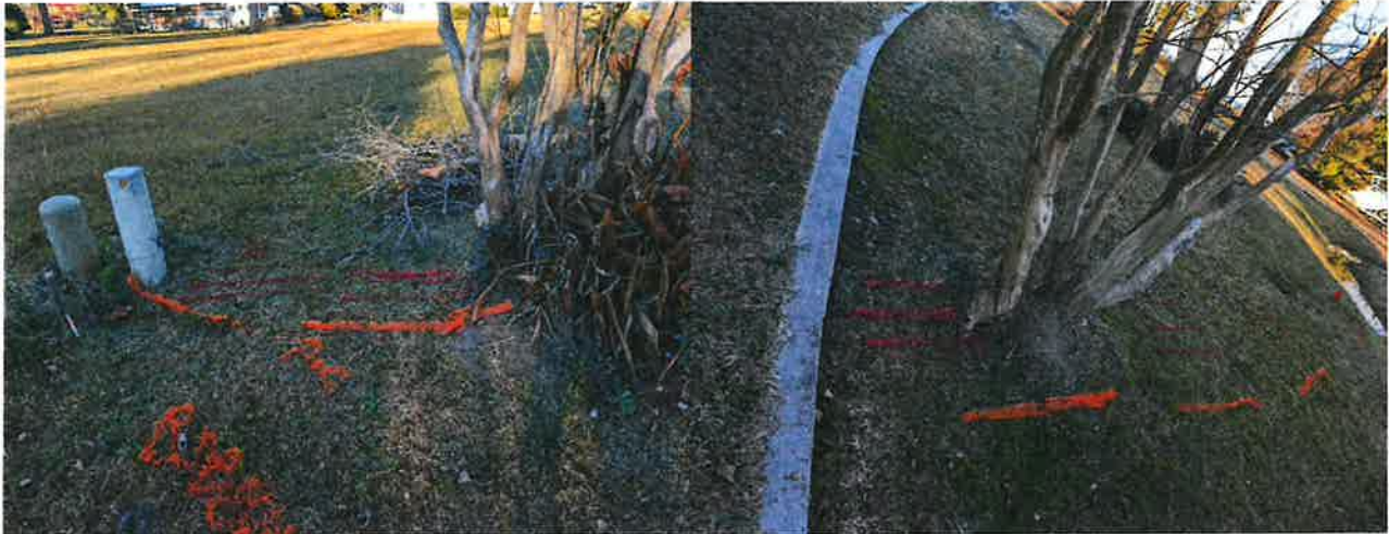
Underground utilities run underneath town crepe myrtle trees Trees have been in place fo a long time with an extensive root system.
