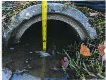
15-16 inch existing concrete pipe
